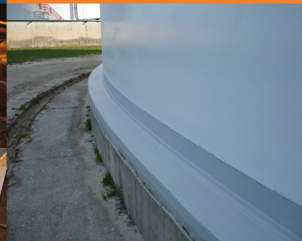
TANK BASE SEALED
