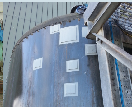
TANK WALL REPAIRED
