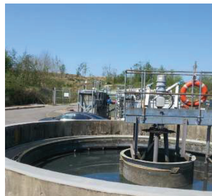
Clarifier rebuilt with Belzona materials providing chemical and impact resistance
