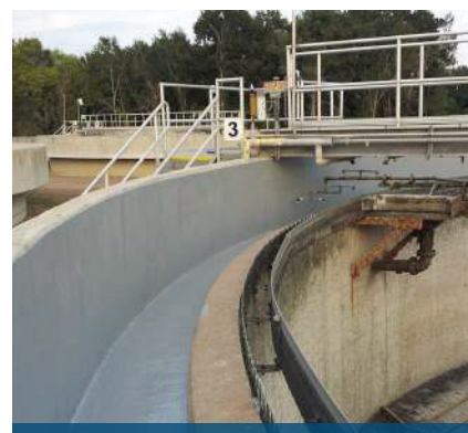
Clarifier rebuild and coated with Belzona materials
