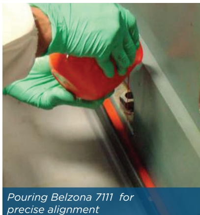
Newly installed equipment requiring chocking
