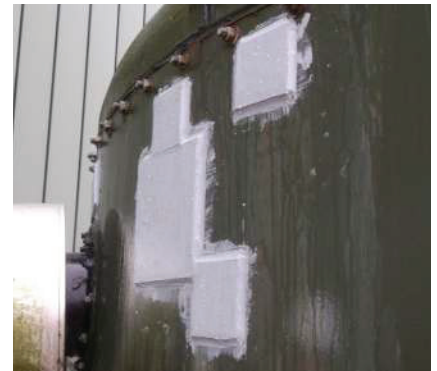
Tank repaired by cold bonding
