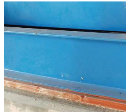
Belzona 100% solids chocking compound applied
