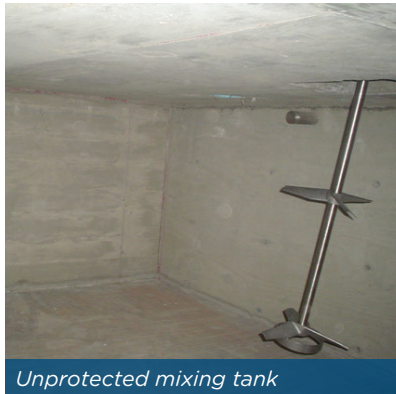
Tank showing severe corrosion
