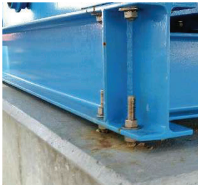
Newly installed equipment requiring chocking
