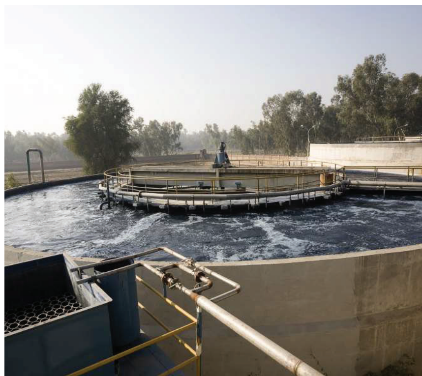
Clarifier repairs completed
