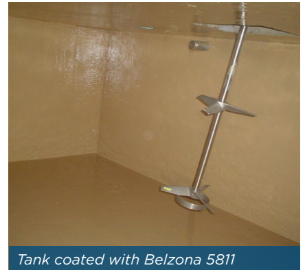
Tank lined with Belzona 5811
