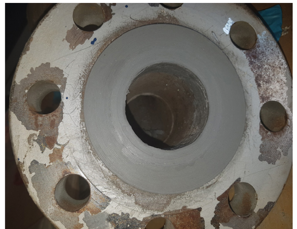
Completed flange face forming repair
