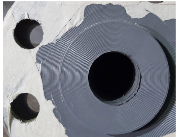
Flange faces rebuilt and restored with Belzona 1111 (Super Metal) using forming technique
