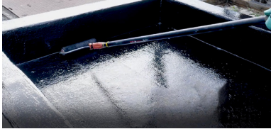
Belzona 5813 Solvent-free, cost-effective static-dissipative barrier coating designed to transfer the build-up of electrostatic charge away from hazardous areas.
