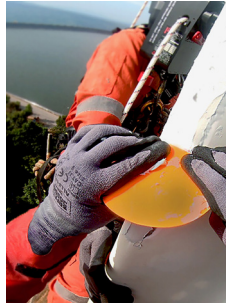
Belzona 5711 High-performance, solvent-free rebuilding material designed for repairing damage to the leading edges of wind turbine blades.
