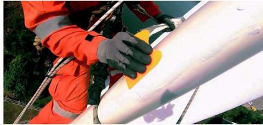
Belzona 5711 High performance, fast curing system for the repair of erosion and impact damage on leading edges of wind turbine blades.
