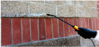
Belzona 5122 (Clear Cladding Concentrate) Breathable, transparent, water-repellent treatment suitable for protecting porous masonry surfaces such as brickwork from water penetration.
