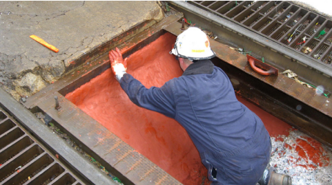
Belzona 4181 (AHR Magma-Quartz) Acid and heat-resistant epoxy concrete repair mortar.
