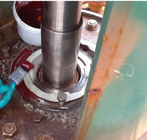
Belzona 4331 (Magma CR3) Epoxy novolac barrier coating for concrete and metal protection, offering high resistance to hot organic acids.
