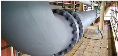
Belzona 5851 (HA-Barrier) Heat-activated, surface-tolerant epoxy coating suitable for protecting hot metallic substrates operating between 70°C (158°F) and 150°C (302°F).
