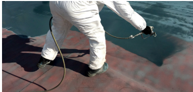
Belzona 6111 (Liquid Anode) Zinc-rich epoxy coating suitable for providing long-term galvanic protection to metallic surfaces.
