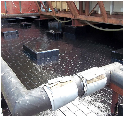
Belzona 4351 (Magma CR5) Epoxy novolac, static-dissipative barrier coating suitable for concrete and metal protection, offering high resistance to a broad range of chemicals.
