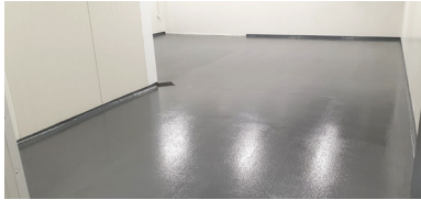
Belzona 5231 (SG Laminate) Chemical and abrasion-resistant, solvent-free epoxy floor coating system suitable for positive grip applications.
