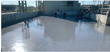
Belzona 5815 Solvent-free, cost-effective flexible coating system suitable for protecting substrates exposed to short-term chemical immersion or spillages.
