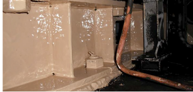
Belzona 5831 (ST-Barrier) Surface-tolerant epoxy coating suitable for the protection of wet, oily and underwater surfaces operating between 5°C (41°F) and 40°C (104°F).
