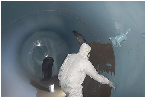
Belzona 1391T Hand-applied, high-temperature, abrasion-resistant epoxy coating for erosion-corrosion protection under immersion up to 130°C (266°F).
