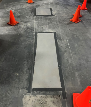
Belzona 4111 (Magma-Quartz) A magma-consistency repair/rebuilding system for repairing and resurfacing concrete and stonework.
