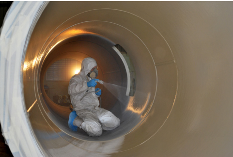
Belzona 1381 Sprayable, erosion-corrosion-resistant epoxy coating with ultra-high molecular weight polymer fillers for immersion up to 95°C (203°F).
