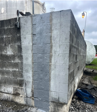
Belzona 4111 (Magma-Quartz) A magma-consistency repair/rebuilding system for repairing and resurfacing concrete and stonework.
