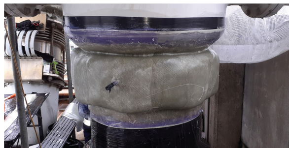
Belzona 7311 applied to breather membrane with Belzona 9341 incorporated. 5x layers of Belzona 9371 utilising Belzona 1981 resin
