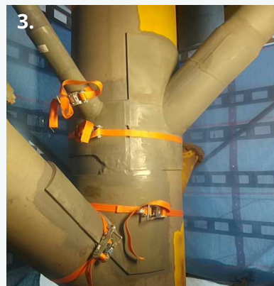
Rebuild and Repair
