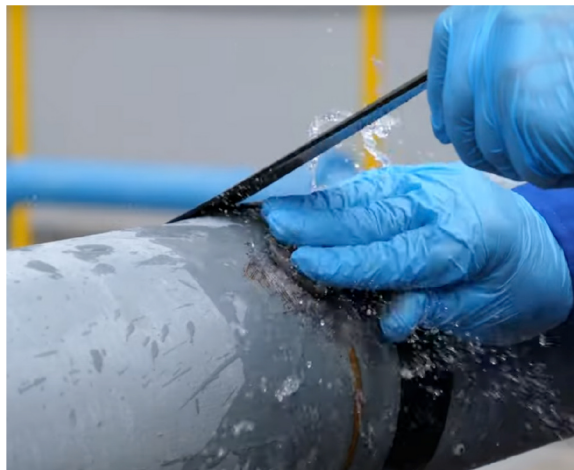
Leak sealed with Belzona 9611
