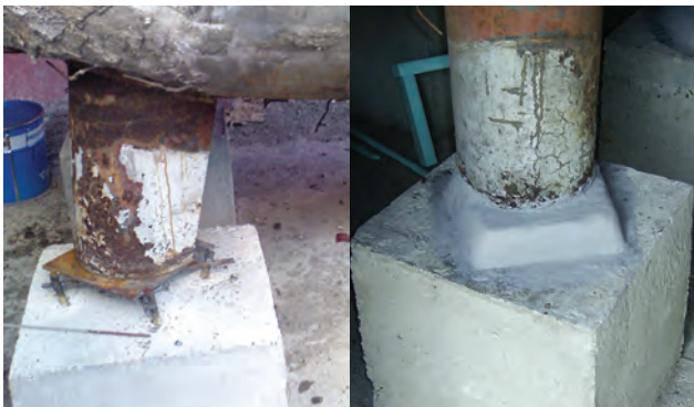
Vessel supports repaired and protected
