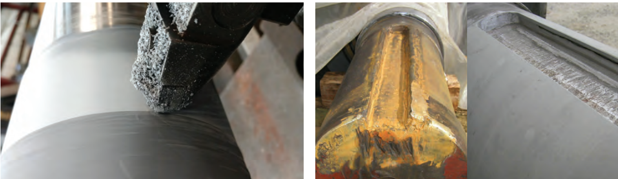
Shaft rebuilt using Belzona paste-grade material Jaw crusher's damaged shaft and keyway repaired
