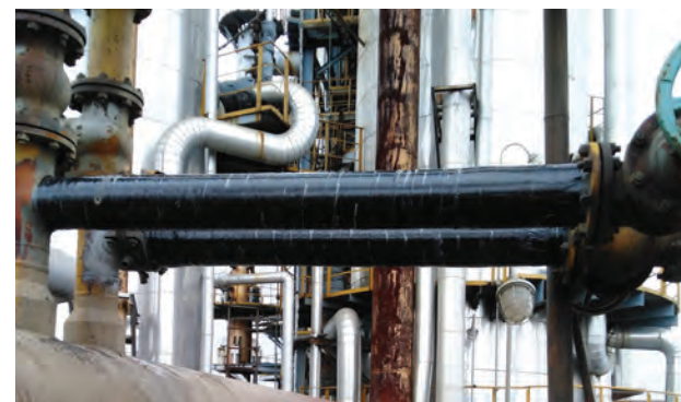
Pipe wall strength restored using compliant pipe wrap
