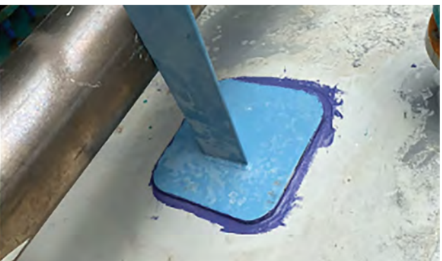
Belzona 7311 bonding pipe supports on the top of a tank
