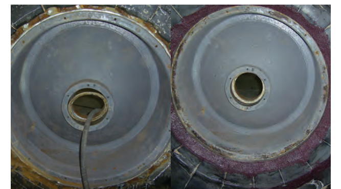
Separator inlet restored
