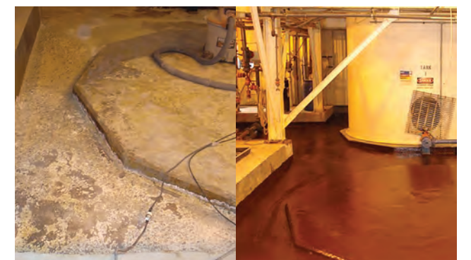
Concrete was rebuilt and protected from sulfuric acid damage
