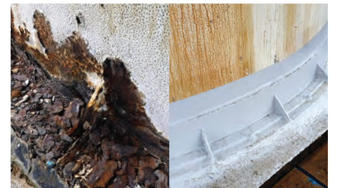
Tank base repaired and restored from corrosion
