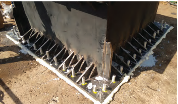
Concrete shimming of crane base
