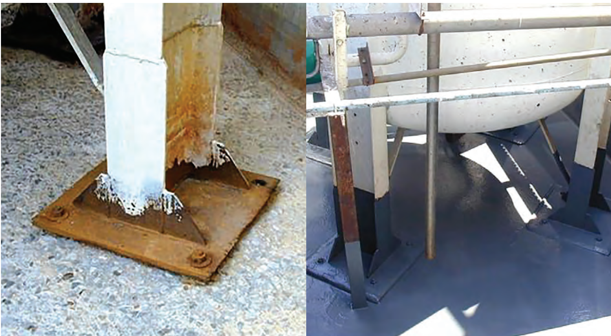
Deterioration of the concrete due to leakage and contamination
