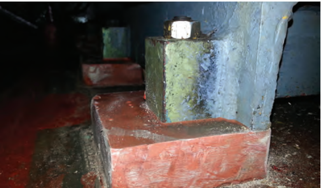
New boiler required chocking into place
