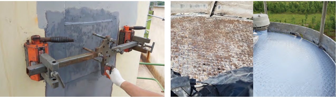
Corroded tank wall repaired Lid repaired with plate bonding technique
