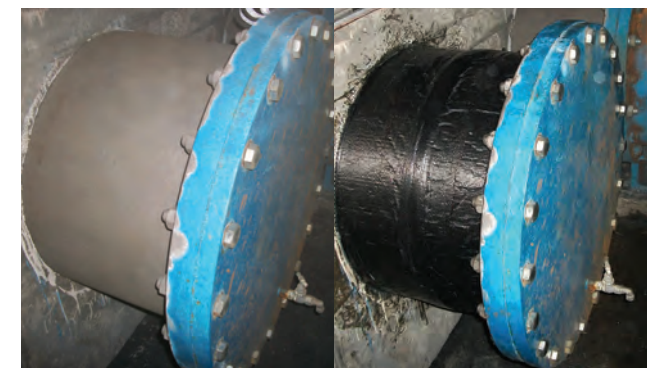
Wrap repair on pipework
