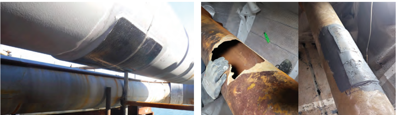
Composite pad installed for pipeline repair Damaged GRP pipe repaired using Belzona's cold bonding solution
