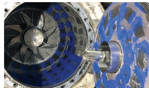
Abrasion resistant grouting repair for turbo separator
