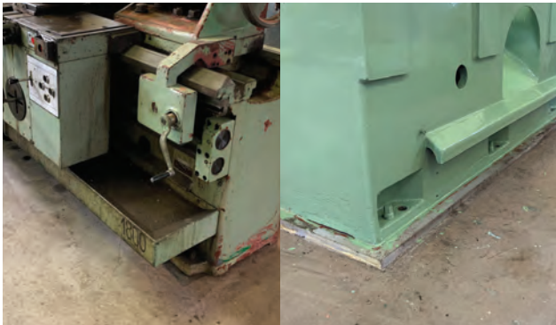
Installed lathe required chocking for stabilization
