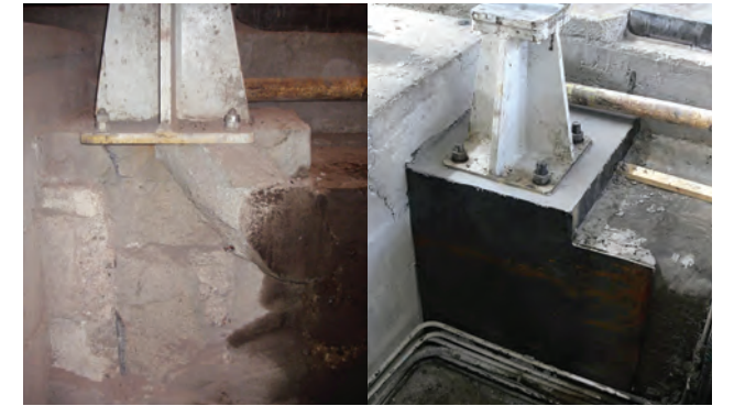
Damaged concrete footing repaired and rebuilt
