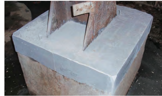
Metallic footing of a pulper and concrete restored
