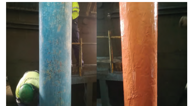
Exposed hot pipeline made safe with insulation
