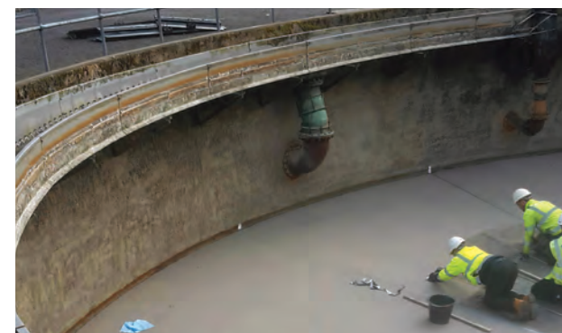
Repair of a large wastewater clarifier suffering erosion and chemical attack
