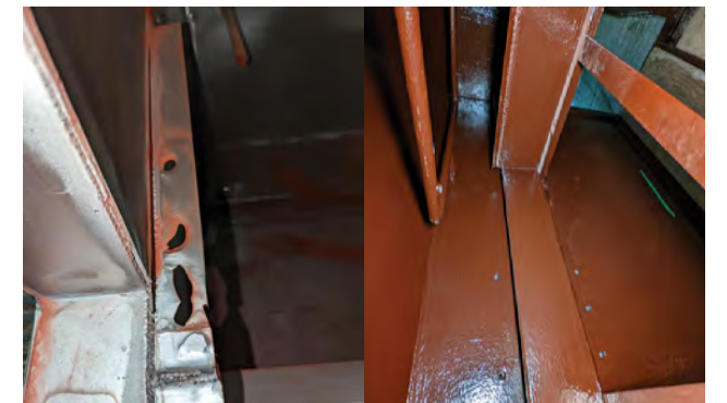
Scrubber vessels coated to protect from chemical attack
