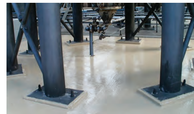
Spirit containment area repaired and protected
