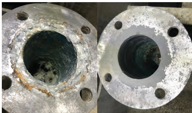
Emergency flange repair
