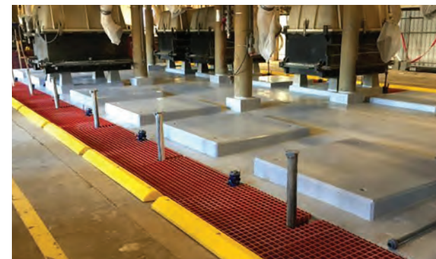
Concrete cell bases rebuilt from chemical attack
