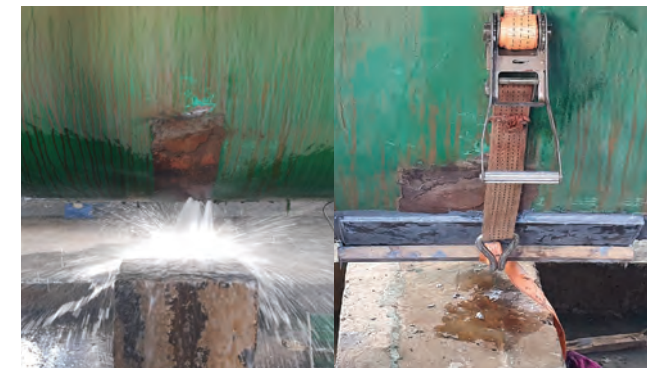
Live leak on a pipe sealed with Belzona
