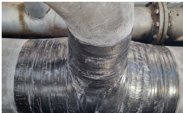
Belzona SuperWrap II Installed at a refinery
