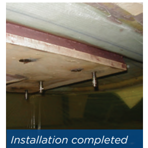
Close up of bonded area
