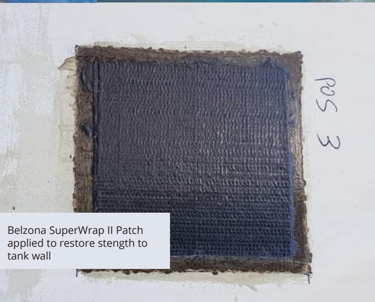
Live leak sealing using plate bonding method
