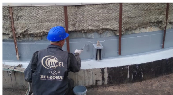
Base of a hydrocarbon storage tank sealed and protected with Belzona.
